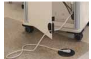
SIDE PANEL POWER CABINET
